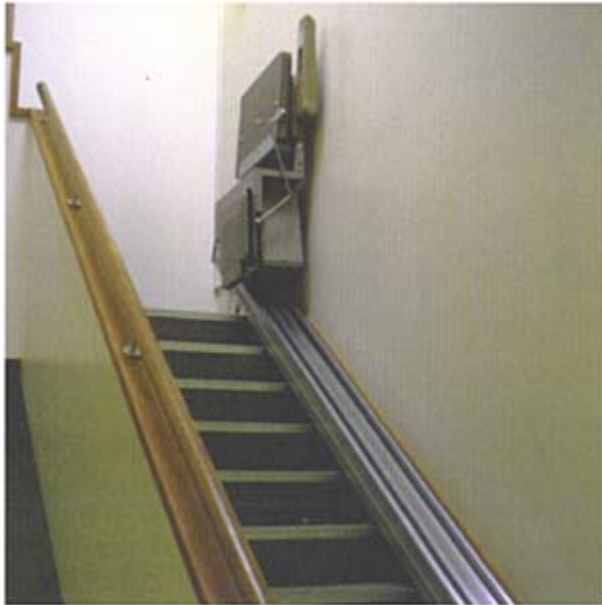
Fig. 5.6.2a: Typical stair-lift installation
