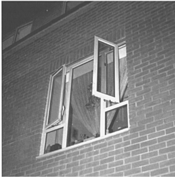
Fig. 5.1.9b: Windows left open at night to dissipate excess heat.
