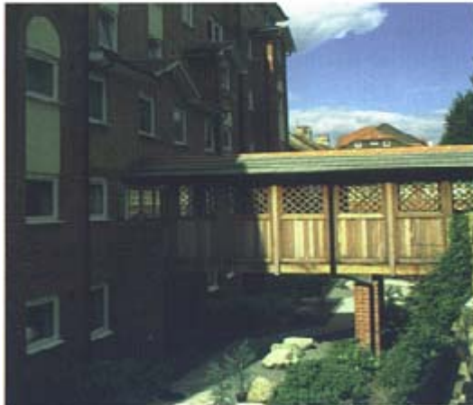
Fig. 1.5.4d: Retirement flats, private development
