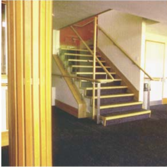
Fig. 4.6.1b: Contrasting nosings and handrails
