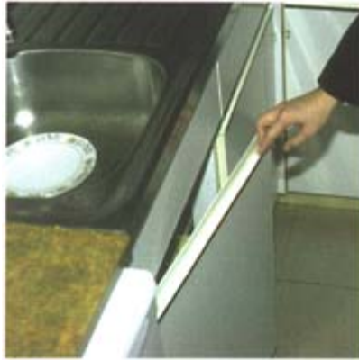
Fig. 4.2.5d: Awkward recessed strip handle
