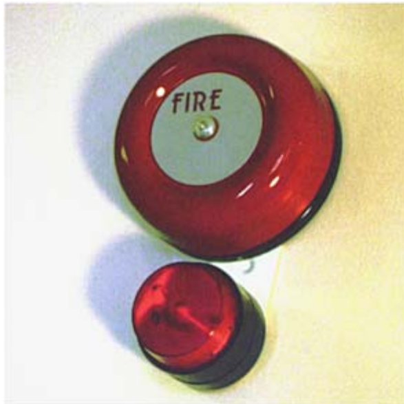
Fig. 5.8.4a: An audible and visual fire alarm
