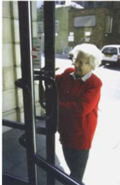
Fig. 4.3.1g: Excessively heavy doors
