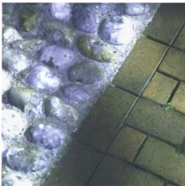
Fig. 2.5.2r: Changes in floor surface
