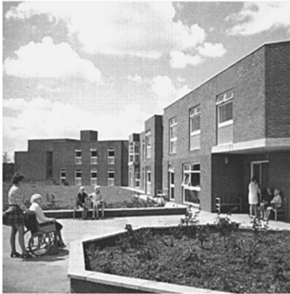
Fig. 1.5.5a: Local authority residential care home
