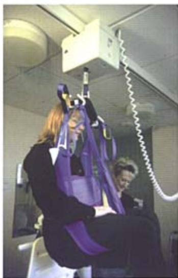
Fig. 5.6.1b: Using a ceiling hoist
